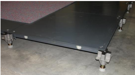
(1) Corner-locking FM-Panels to FM-Pedestals
