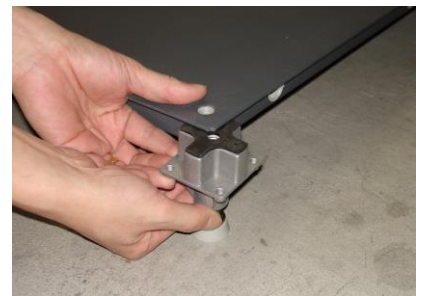
(3) install FM-pedestal at field
