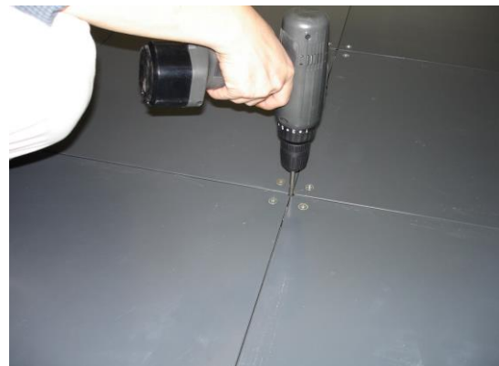
(4) Hexagon key-wrench fastening from top by mechanical tool
