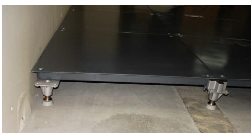
(6) FR-pedestal installed at perimeter
