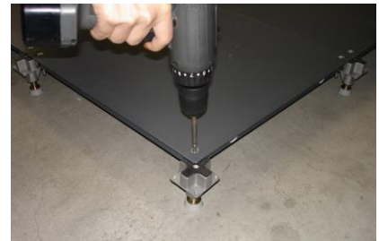
(1) Corner lock access panels onto pedestal headset by mechanical tool
