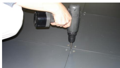
(7) Last step to fasten by 6 mm hexagon key wrench
