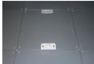
cut carpet for single FM-lid exits up to 5 ~ 6 data wires
