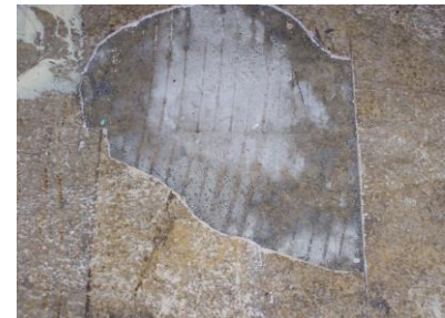
The adhesives damage sub-floors when removing pedestals
