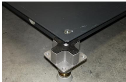
(1) Corner lock access panels onto pedestal headset by mechanical tool
